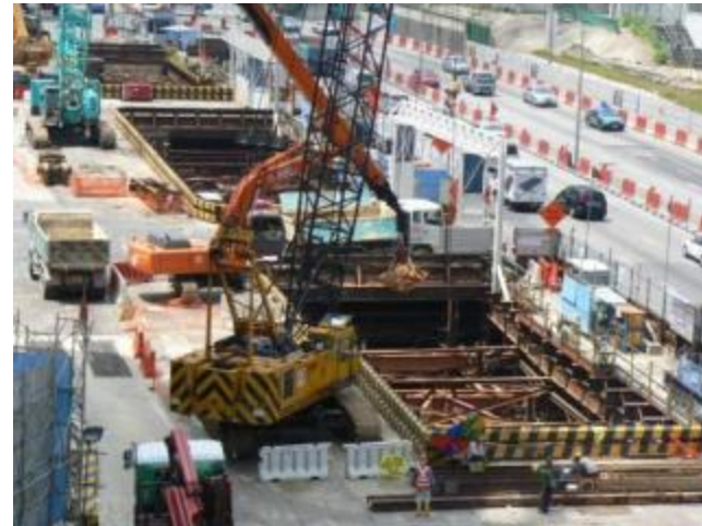
Farrer Station, Circle Line, Singapore
