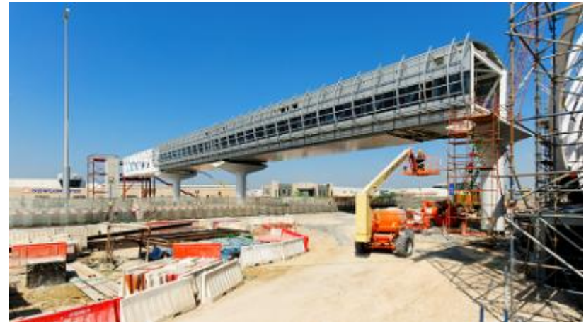
Dubai Metro Rail, Dubai
